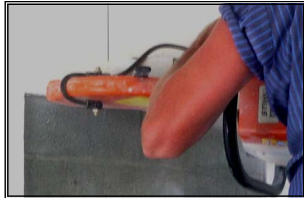
Fig 4. Saw Between the Holes
