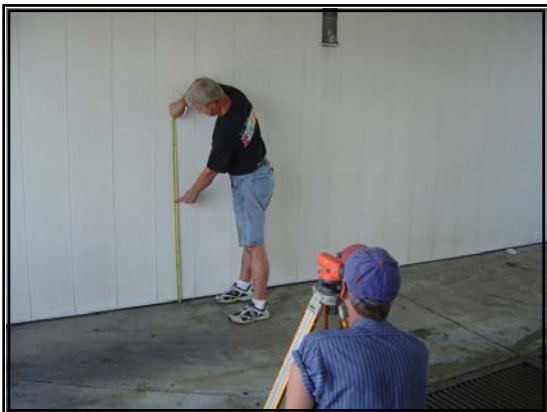
Fig 1. Mark 3 Level Points on Each Wall
