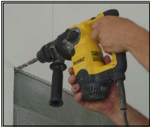
Fig 3. Hammer Drill the Corners
